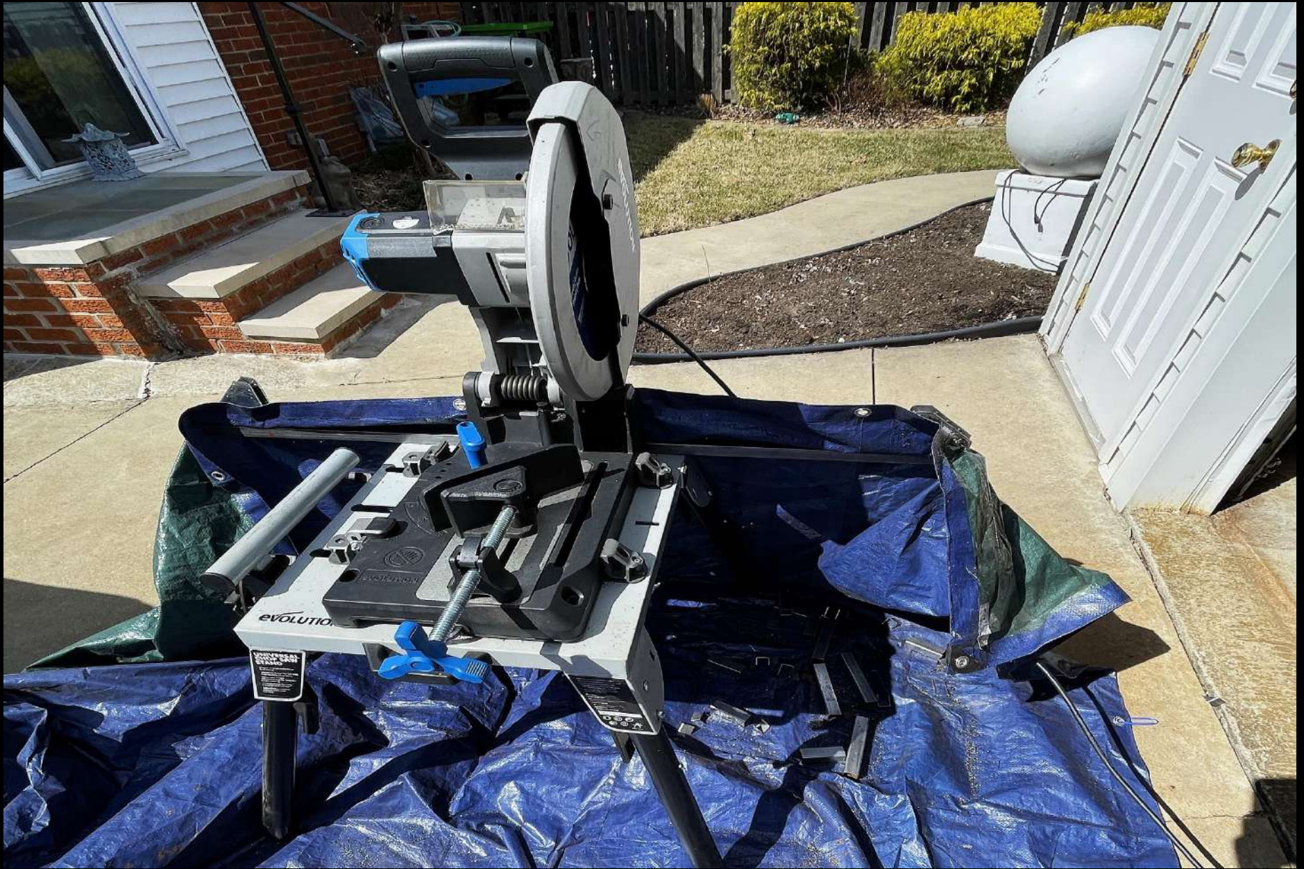
The steel chop saw is set up to make the 45-degree angle miter cuts for the fountain flutes, the fountain vertical legs and on the top cross rail.
