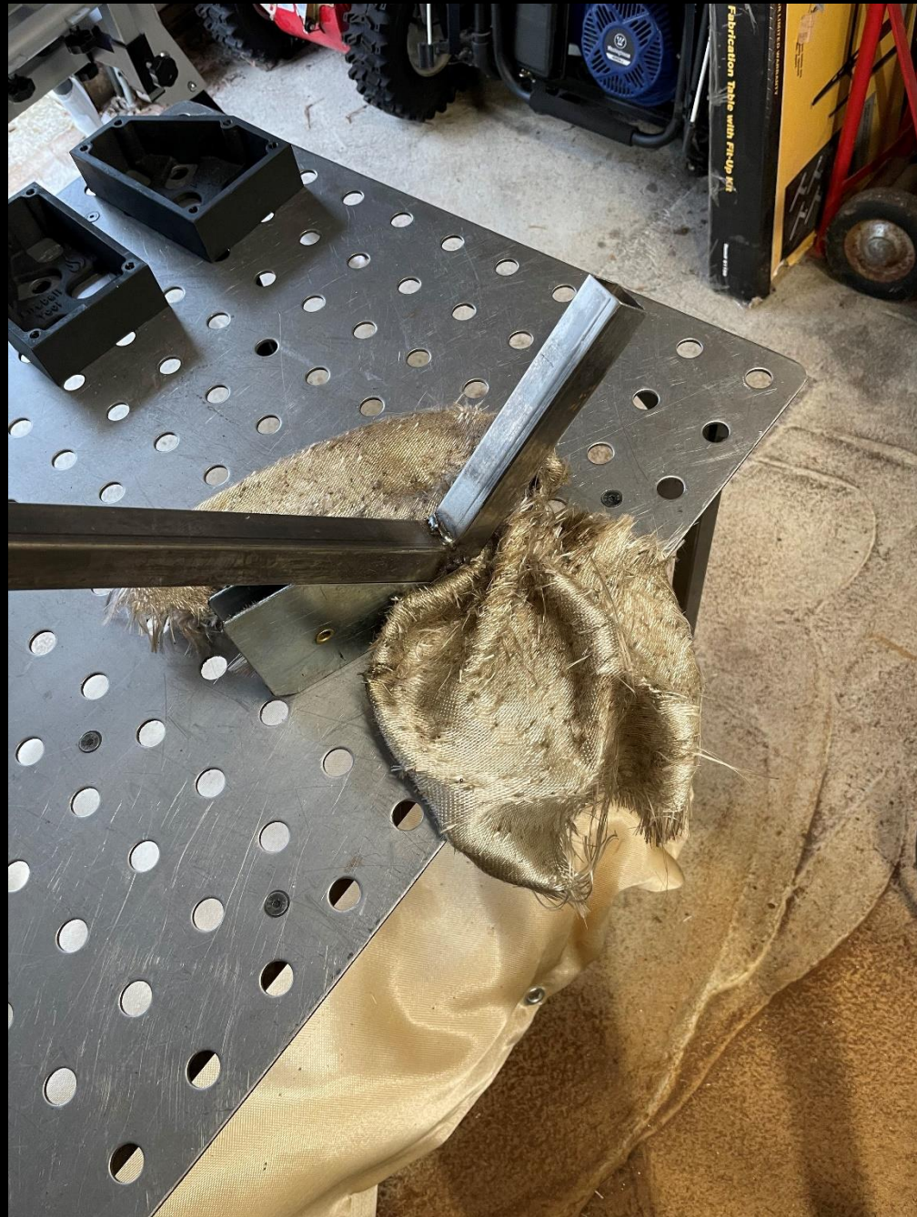
Spa Book Shelf- Fabrication Sequence: 7 Using 45 degree angle on welding magnet.
