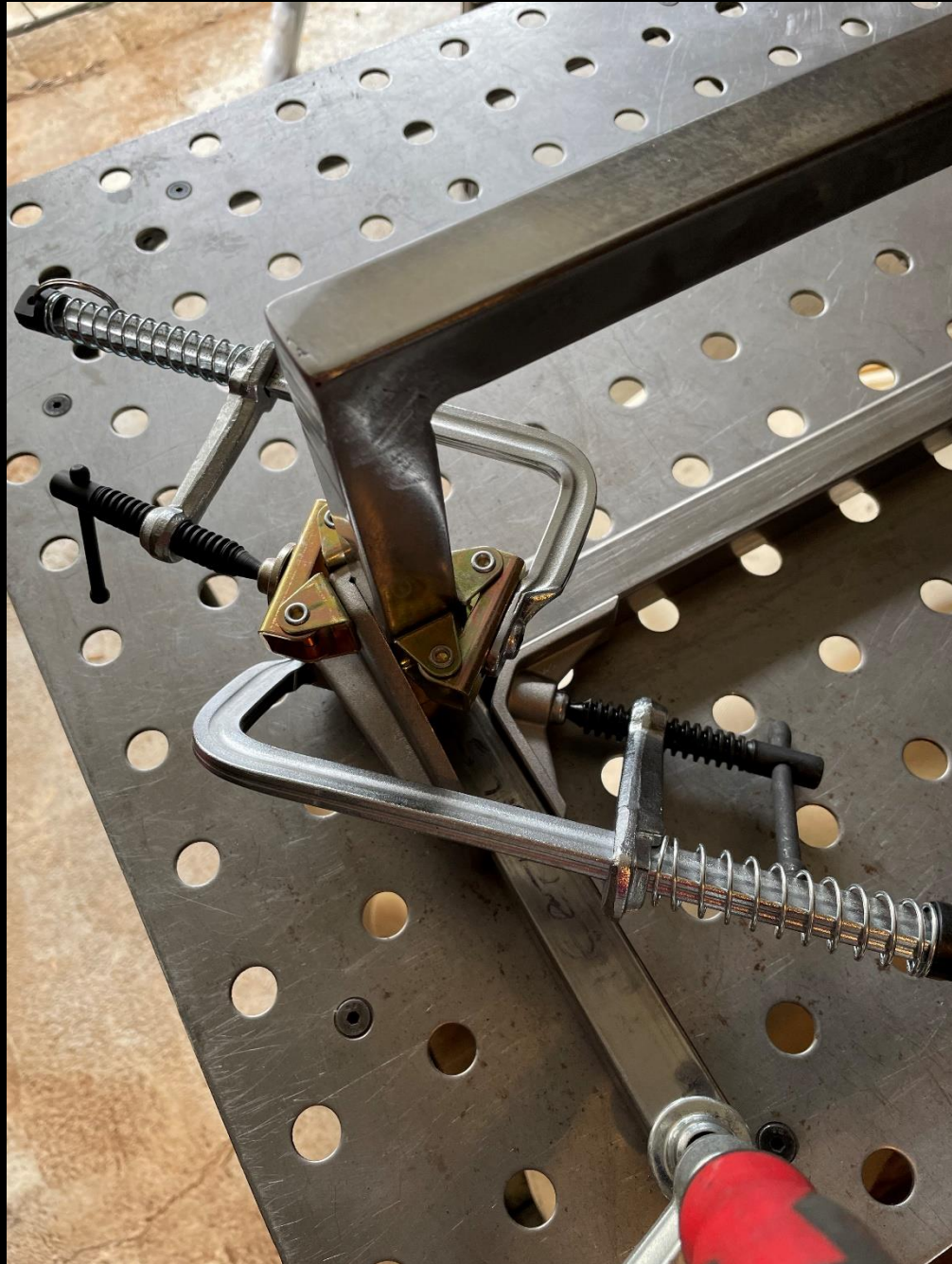
Spa Book Shelf- Fabrication Sequence: 20 Tack weld upper shelf and back-side B.
