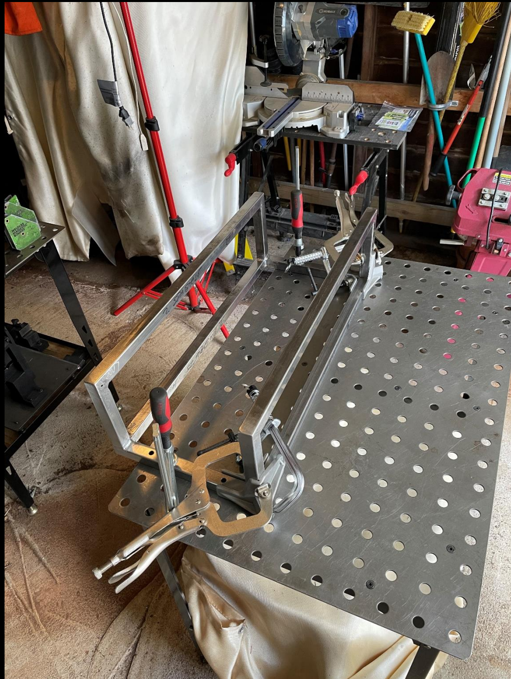
Spa Book Shelf- Fabrication Sequence: 18 Weld upper shelf to vertical legs & back.
