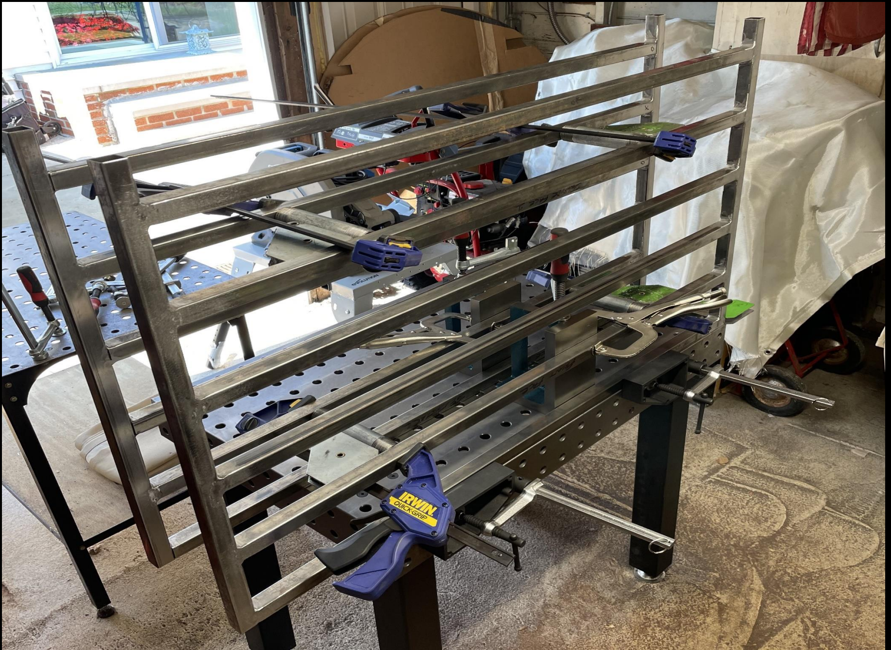
Sedona Wine Rack #12 Fabrication Sequence: 10 Panels 1 and 2 can now be welded
